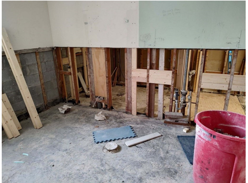
Demolition of bathrooms
